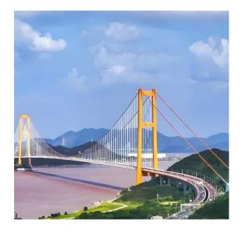
We supplied 28,500 tons of Q345C steel plates, 6,300 tons of Q345C coils, 6,200 tons of steel wires and galvanized steel wires, 9,400 tons of steel strands, and 22,800 tons of rebar, all meeting the 1770 MPa strength level with outstanding corrosion resistance and weldability to ensure structural stability and durability.
